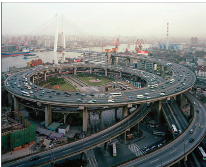
Obr. 26: Edward Burtynsky, Nanpu Bridge Interchange, Shanghai, 2004
