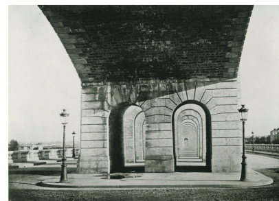
August Collard, Viaduct , asi 1870
